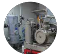
Pressure testing of components
