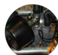
Inlet Blower Filters
