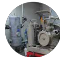
Pressure testing of components
