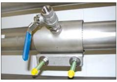
If there is no measuring site with 1/2" ball valve present it can be set up by means of spot drilling collars
