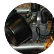
Inlet blower filters
