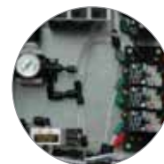
Pneumatic control systems
